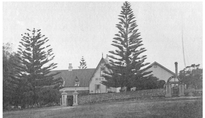
The pre-fire Isle of Wight Hotel. Looking across paddock towards hotel with gabled roof and dormer windows, arched sign over entrance gate reads: Isle of Wight Hotel, wooden railing fences in right foreground and on left, bordering road towards hotel. Source: State Library of Victoria. H33027/21d.
