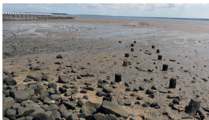
The Grantville piers, old and (relatively) new in 2020.
