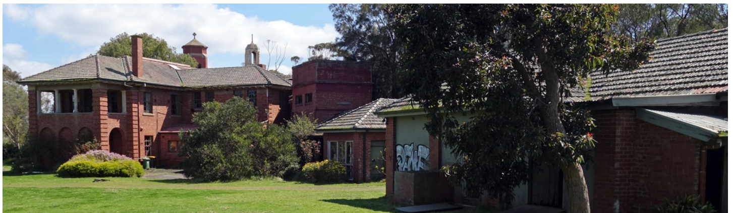
A 2019 photographs of the long abandoned and now decaying and much vandalised St. Paul's Home for Boys.
