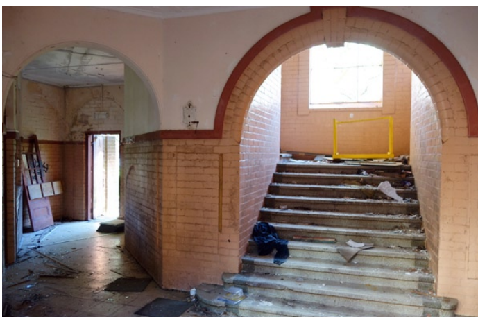
Stairs to 2nd floor dormitories in one of the main buildings.
