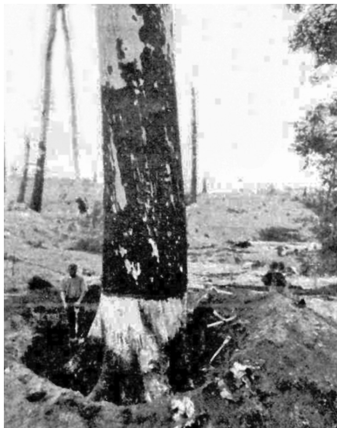
Grubbing a dead giant. Source: the Leader , Saturday 20 August 1910, page 27: Wonthaggi Water Supply. Photo by Vallan Studio, Mansfield.
