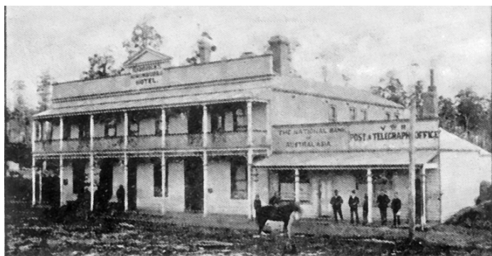
Radovick's Hotel, the bank and the post office. From the Illustrated Australian News , 1 May 1893: Views around Korumburra.
