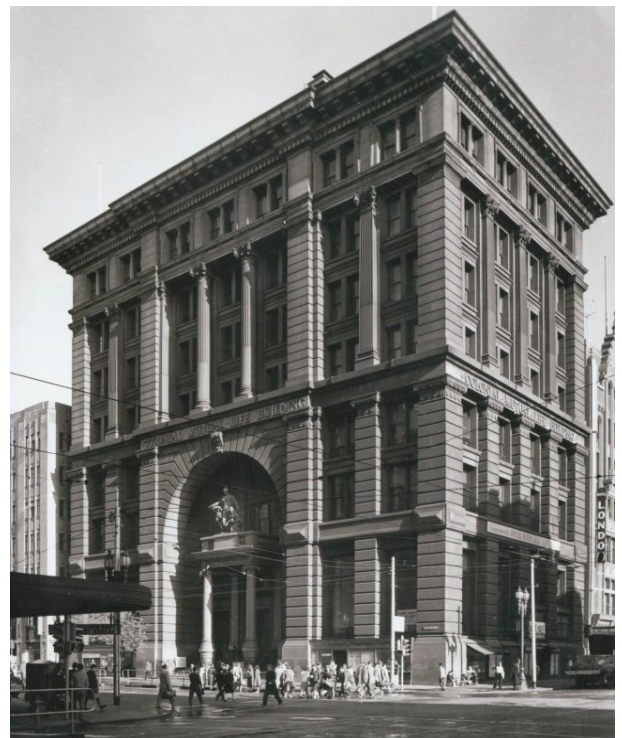
The Equitable Building, corner of Collins and Elizabeth Street, in the 1950s. It was designed about 1890, and took 6 years to build, constructed from granite (some of it sourced from the quarry at Cape Woolamai) thick brick walls and a steel frame. It was demolished in 1959.
