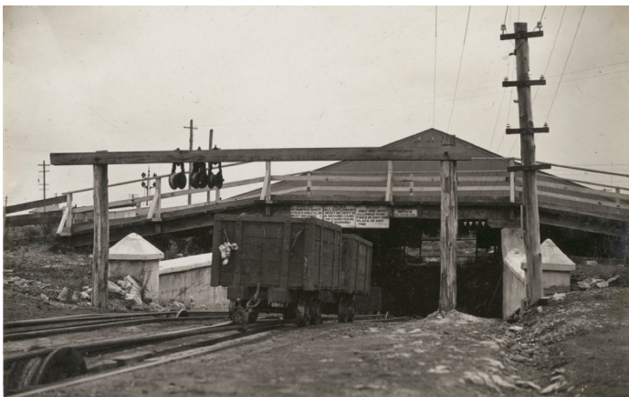
Above: Entrance to McBride tunnel, State Coal Mine, March 1929, showing mine entrance with tracks carrying coal trucks running into mine; notices above mine entrance regarding explosives. Photo: State Library of Victoria. Donated by Roger Mulligan via the Dept. of Infrastructure, 2006.
