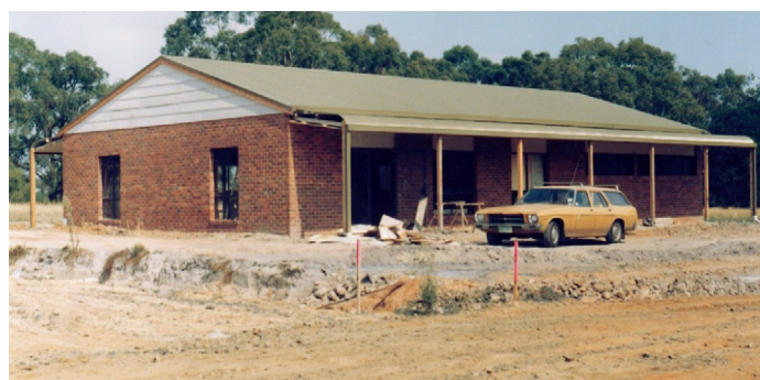
The new Grantville Hall on 23 March 1990.
