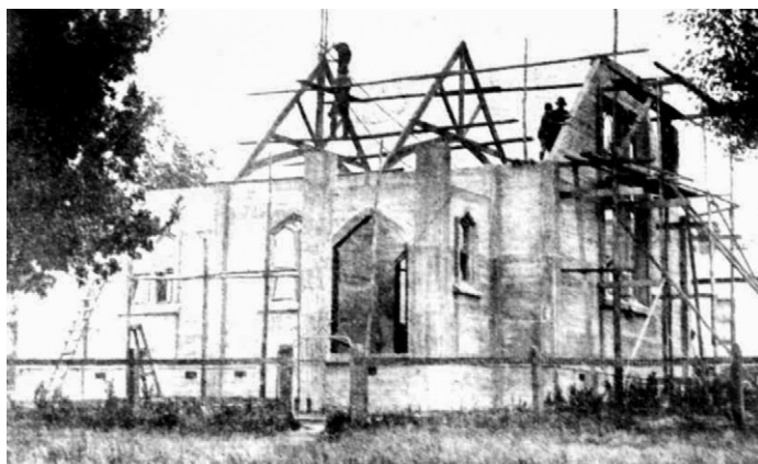
Building a new church of England.
