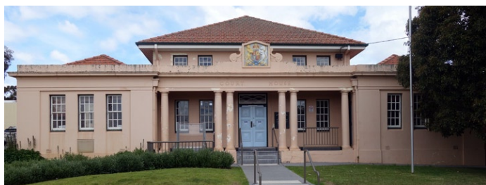
The "new" courthouse in November 2019.
