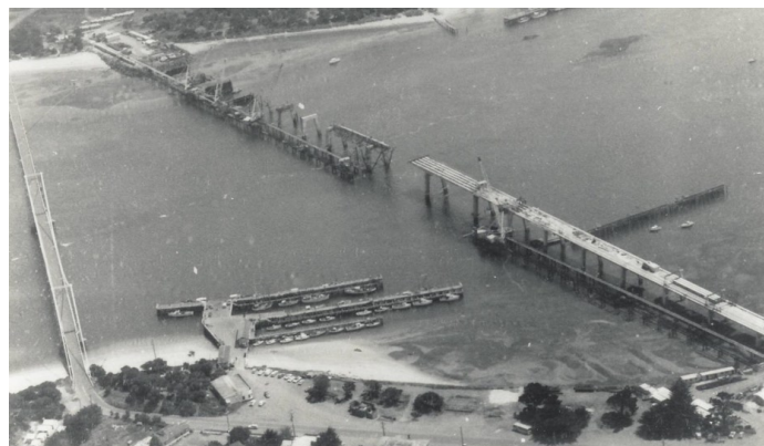
Old suspension bridge on left. The 1969 bridge with all pillars in and decking only partly completed (on right). Source: Jack Jenner collection. Victorian Collections. https://victoriancollections.net.au/items/5600cc82400d0c22a881b58a
